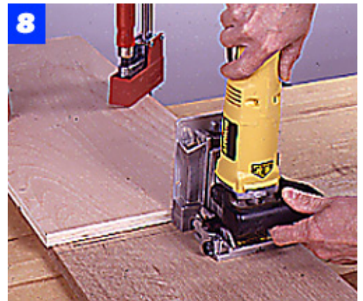
Cut plate slots in the case top and bottom for the partition. Clamp a guide board in place to align the plate joiner.
